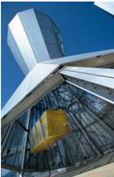
The Sound Tower from outside
