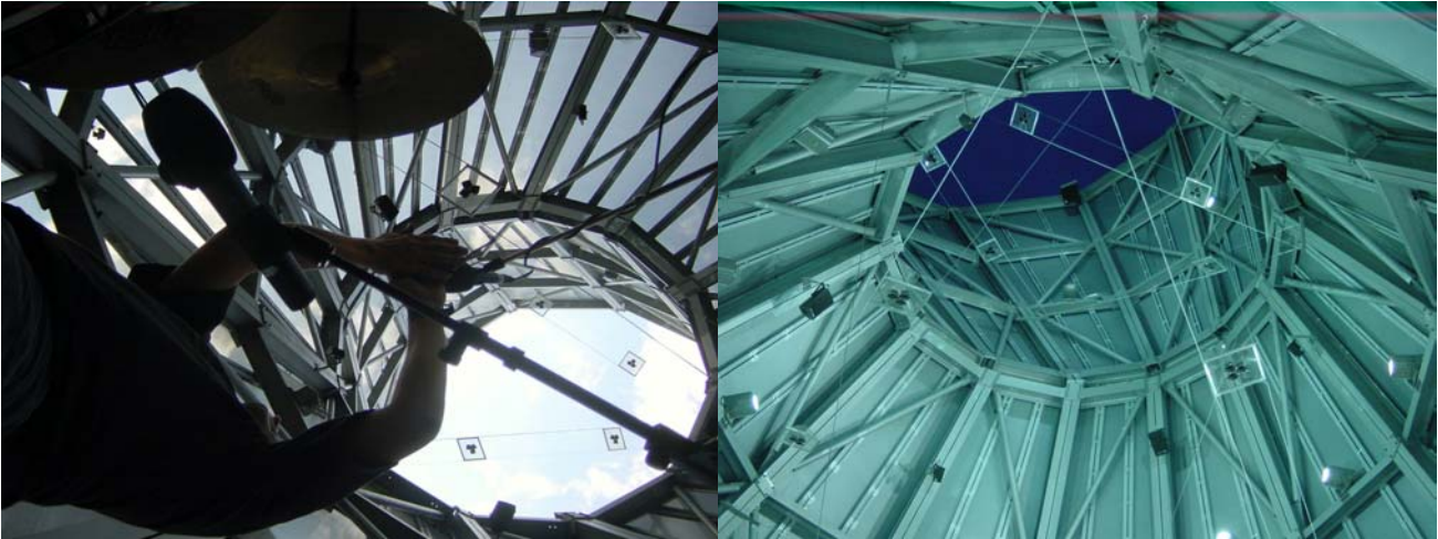
two views from inside the tower towards the sky
